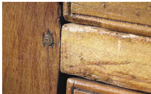
This detail shows the head of a nail driven through a mortise-and-tenon joint.
