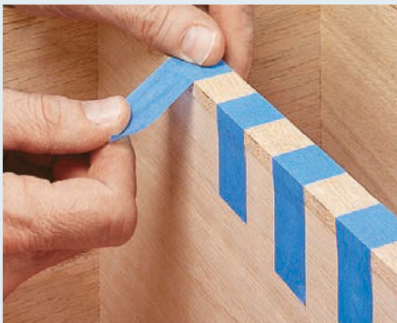
▲ Strips of painter's tape can hold the edging tight while the glue dries. It's a great solution where your clamps won't reach.
